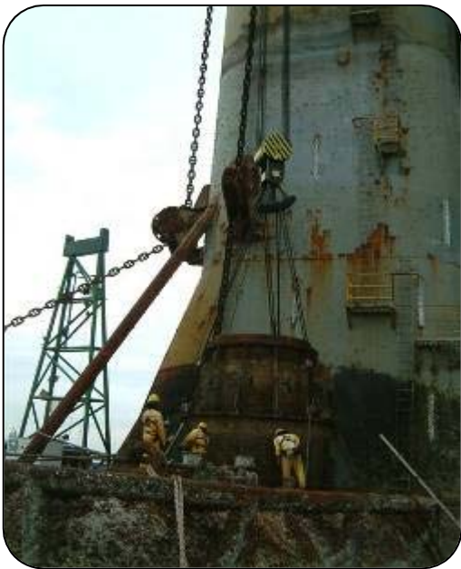
Lifting of Thruster Unit
