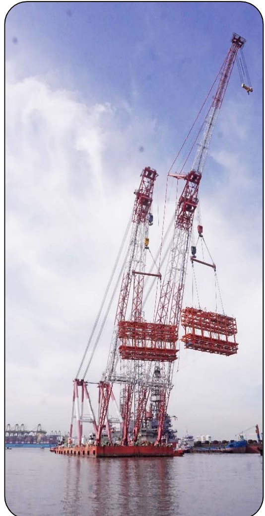
Lifting of pipe racks from yard after completion
