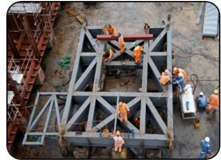
Assembly of Tension Deck
