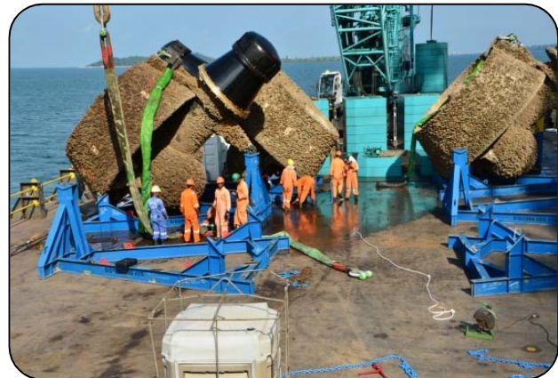
Lifting of Thruster units and loading on Kim Heng 55 Crane Barge
