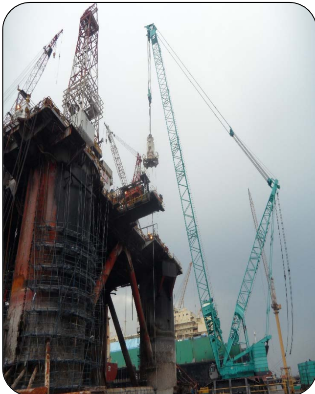
Kim Heng 55 Crane Barge Lifting of LMRP & BOP Assembly from Rig
